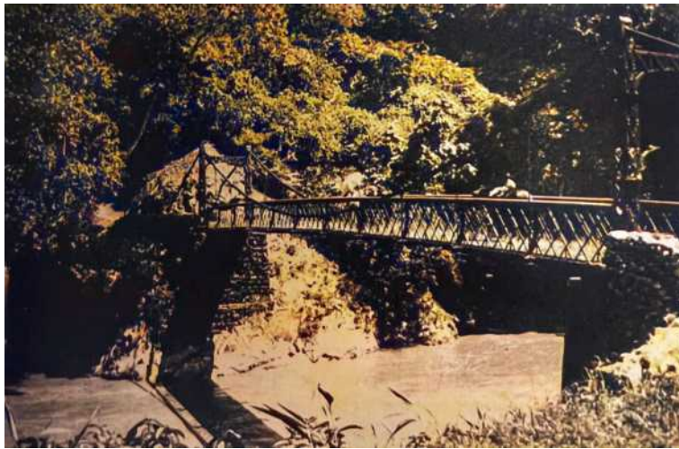
Figure A3: British-constructed bridge across the Doyang river taken by Connie Shakespear, 1900-1902.
